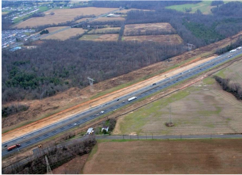
Figure 2.5-2: Construction of Additional Travel Lanes
