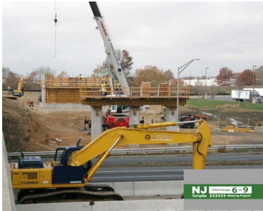
Figure 2.5-3: Bridge Construction over Turnpike
