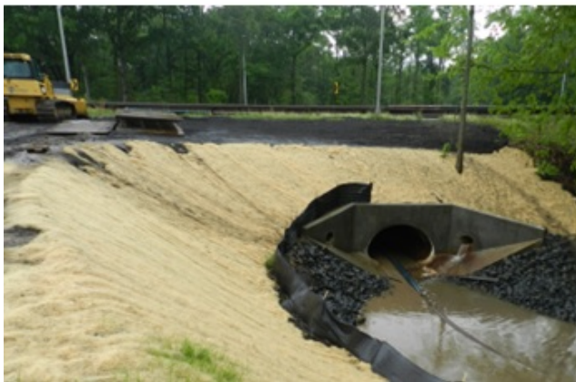
Figure 6: Passaic River Bridges, 16W Ramp Replacement, Parkway Interchange 100 Culvert Rehab
